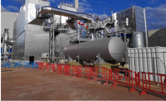
Image 4: The state-of-the-art filtration system in Boffalora sopra Ticino keeps up with the size of the production facilities – and is expected to noticeably reduce dust and nitrogen oxide emissions.
