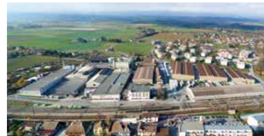
St-Prex Plant Switzerland
