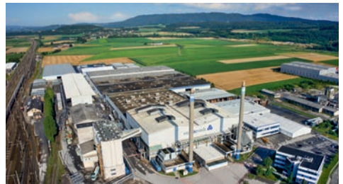
Pöchlarn Plant, Austria
