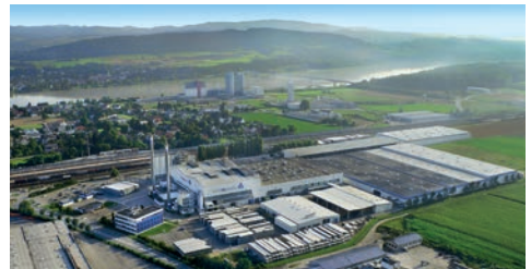
Pöchlarn Plant, Austria
