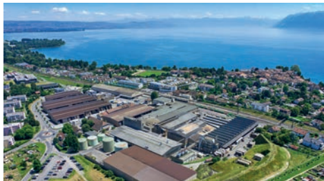
St-Prex Plant, Switzerland
