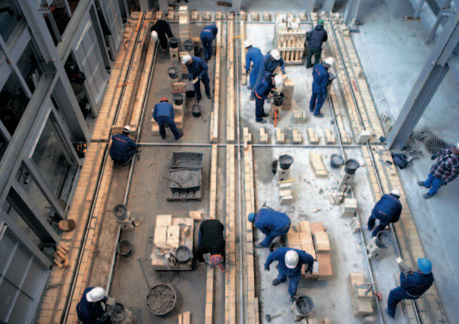
Constructing of the regenerators at the St-Prex facility (Switzerland)
