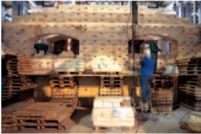
The new green glass furnace in St-Prex (Switzerland) meets the highest standards in terms of energy efficiency and ecology.
