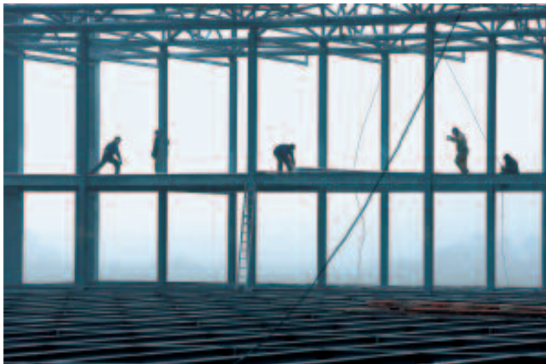
In Gostomel (Ukraine) a new production building for the 380 ton melting furnace is under construction.
