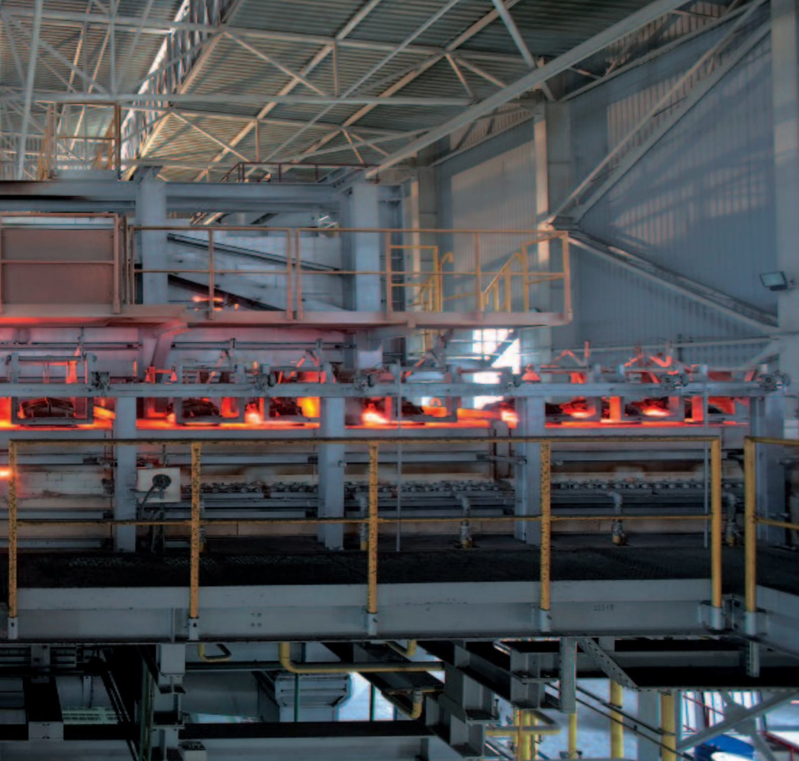
Vetropack Gostomel: New Melting Furnace
