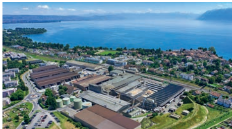
St-Prex Plant, Switzerland
